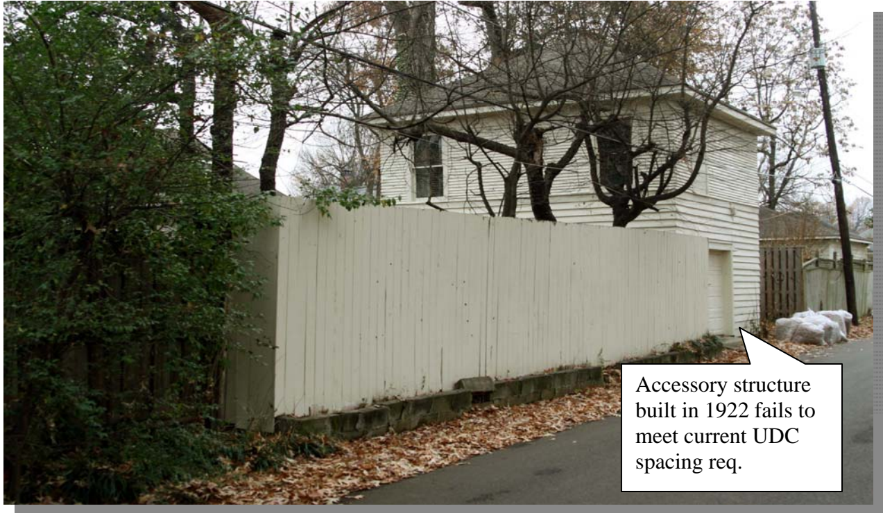
Williamson frontage of accessory structure
