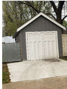
Proposed batten siding color (picture taken up the street from 425 Stonewall).
