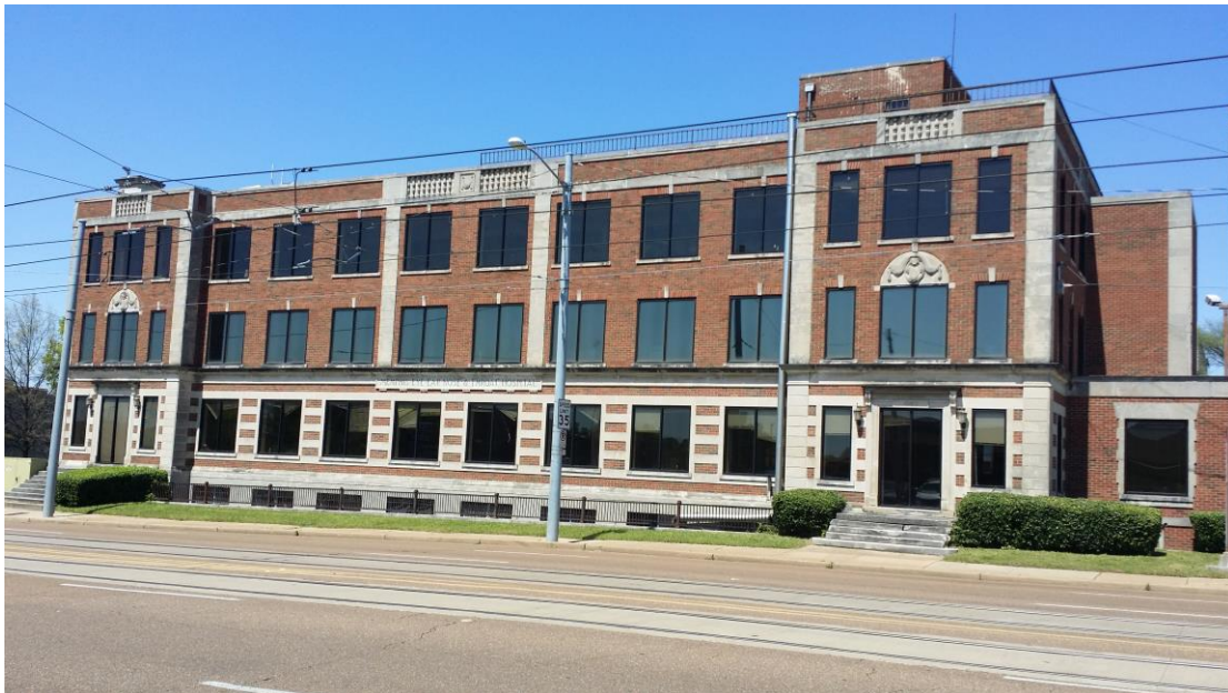
The former Forensics Building at 1060 Madison is being restored to serve as the new location for Community Services Crime Victims Center.
